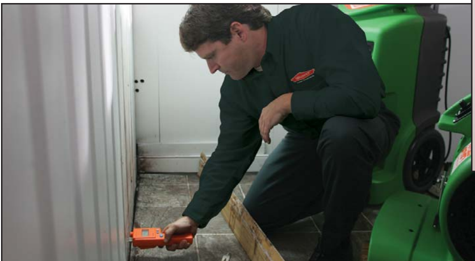
SERVPRO® Professional using a Moisture Sensor and Thermal Camera to detect moisture.
